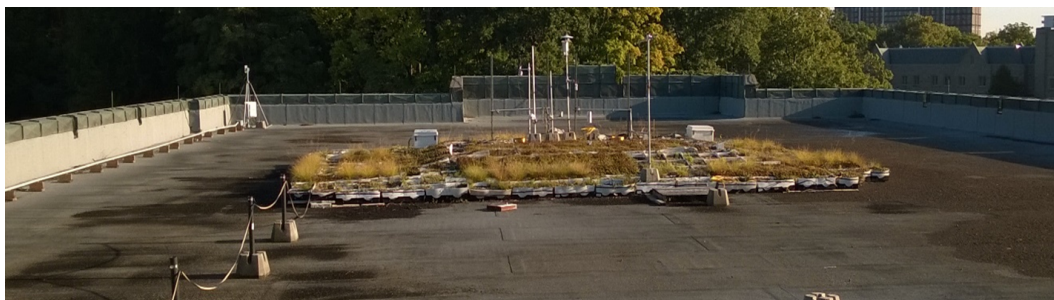
Figure 1. The green roof test array on Talbot College at Western University. Photo credit: J. Voogt.
